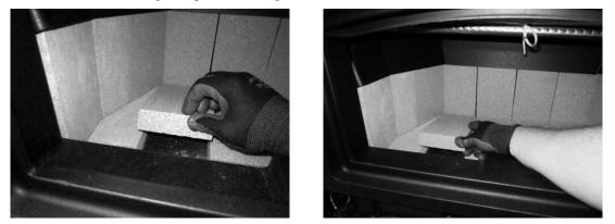
Install the igniter firebrick as shown below. The igniter firebrick has a special hole drilled in it that the igniter will penetrate. Replace the 2 removed floor firebricks.
