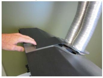
Secure the vent connector to the insert using the screw removed earlier.
