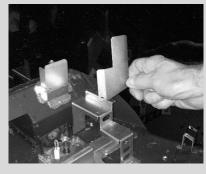
Fit Panel Spacers to the top <u>and</u> bottom edges of the rear fireback panel. There are tabs approximately 1/3 of the way in from each end of the spacer. Place the spacer in the center of the bottom edge of the glass panel. Use your fingers to bend the tabs into a "C" shape around the edge of the glass. Once this step is complete, set the panel aside for installation in a later step.
