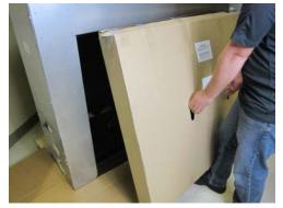
2. Locate and remove the glass frame tool from the fireplace.
