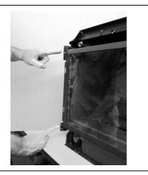
5. Attach the face bracket to the hinge bracket as shown below. The screws insert through the holes in both brackets.
