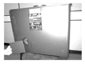
3. Remove the convection chamber cover plate and gasket, as shown below. Retain the screws and gasket.
