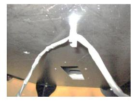
11. Push any excess start switch wiring into the compressor assembly. NOTE: A lock-tie is included to secure excess wiring.
