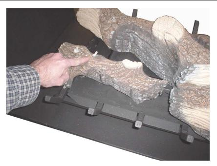
The front left upper log has a groove and one hole on the bottom. The groove fits over the edge of the burner.
