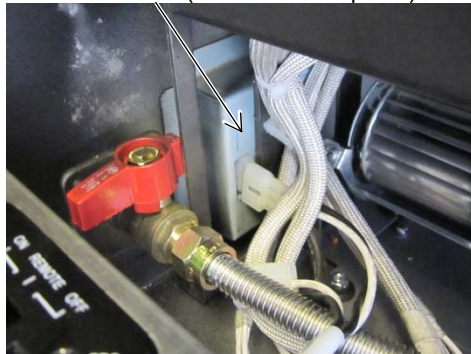
Junction Box (from inside fireplace)
