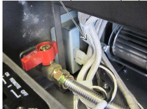
Junction Box (from inside fireplace)
