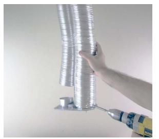
6. Attach the 3" intake vent to the connector and secure with at least 3 screws.
