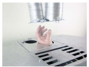
8. Slide the vent connector into place, making sure it fits underneath the tab on top of the insert (see step 3 above for additional photos). Continue to pull down on the connector until it is fully seated.
